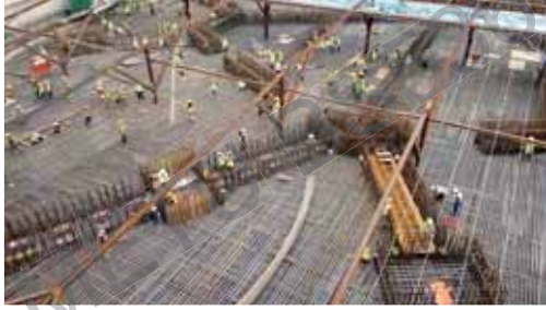
Figure 15 [1] : Core Reinforcement
